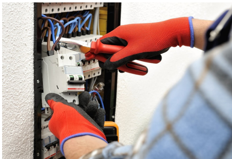
Fig. 4.2.35 Maintaining the electrical integrity of construction equipment
