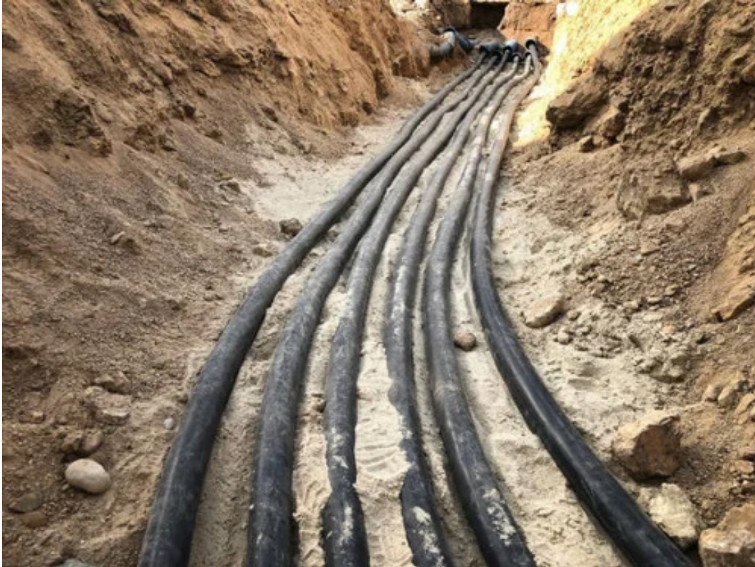
Fig. 3.1.23 Preparatory activities for cable laying
