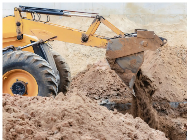
Fig. 3.2.6 Checking trench depth and backfilling
