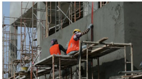
Fig. 1.1.10 Plastering Work
