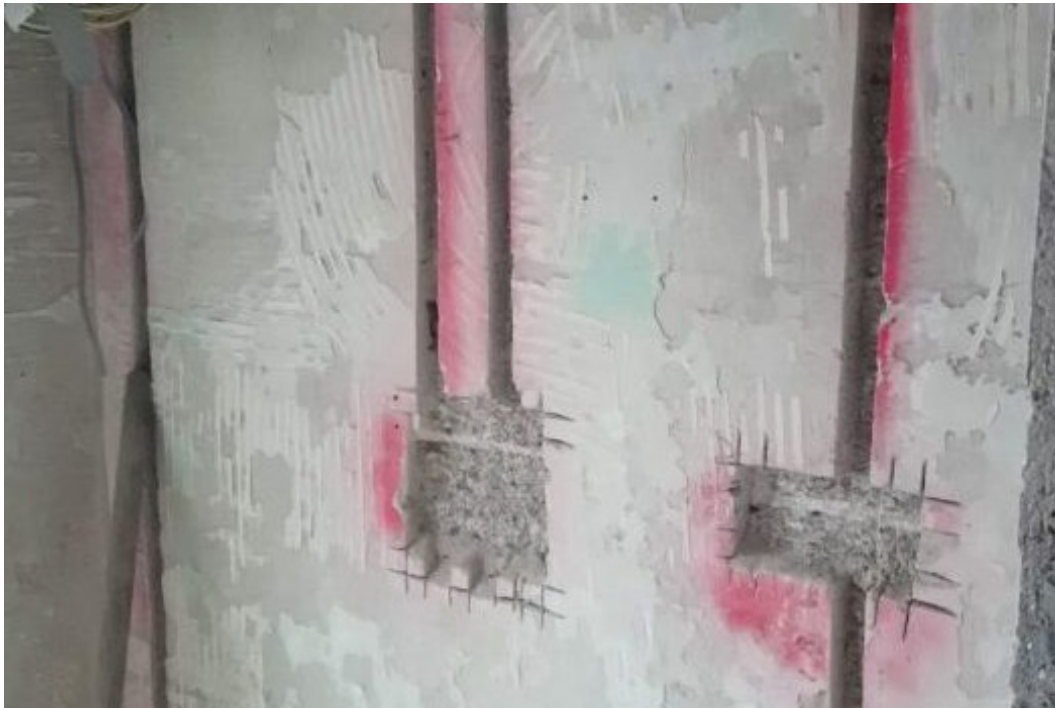
Fig. 5.2.9 Marking the walls for chasing
