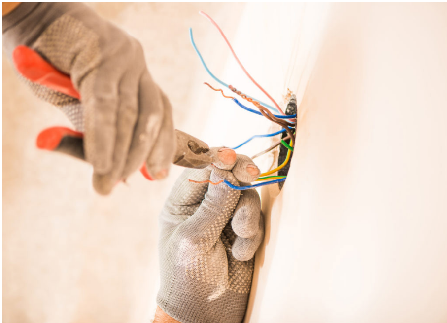
Fig. 4.2.16 Replacement of faulty wiring
