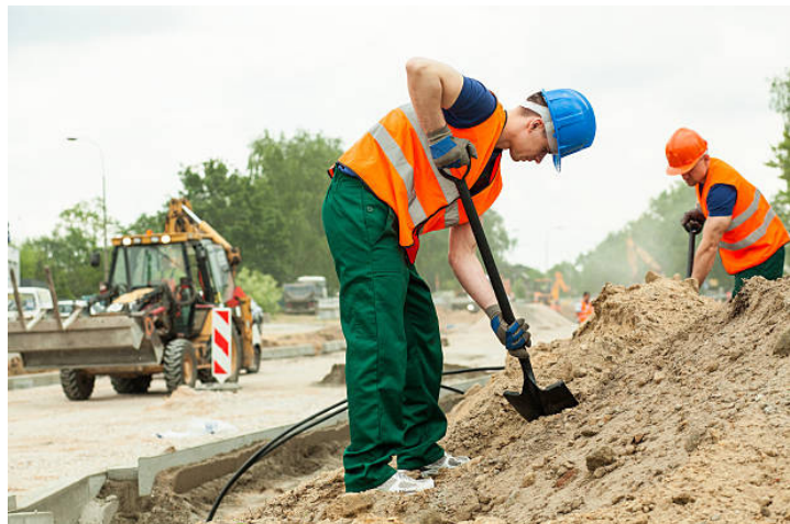
Fig. 3.1.22 Cable laying activity
