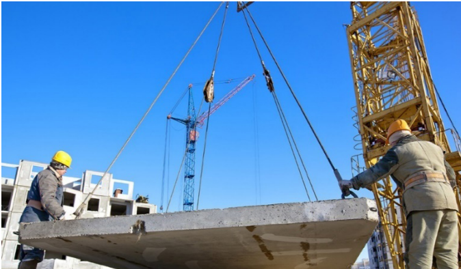
Fig. 1.1.17 Rigging work at site
