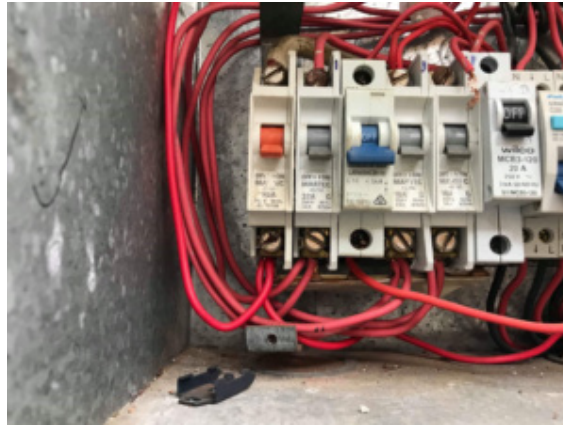
Fig. 3.3.46 Circuit breaker installation
