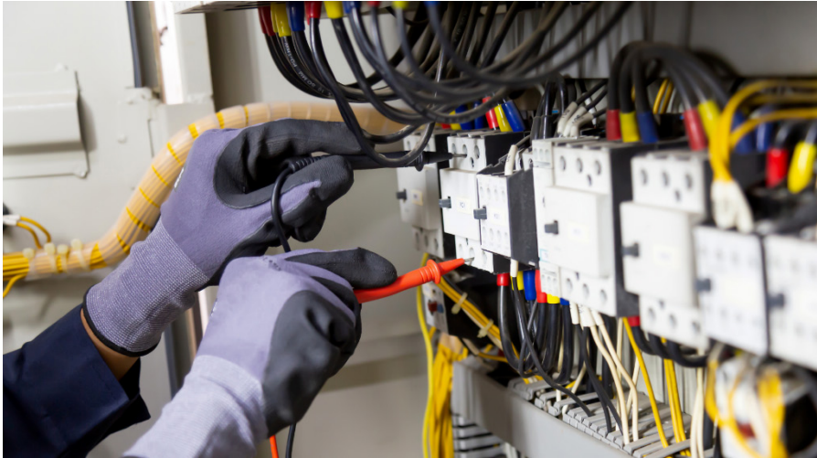
Fig. 3.3.6 Safe work practices
