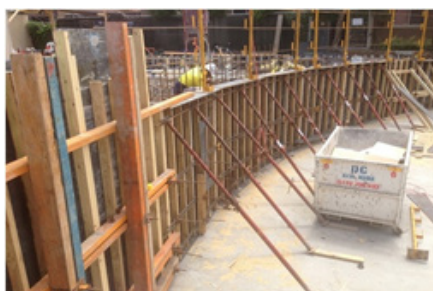
Fig. 1.1.13 Conventional formwork
