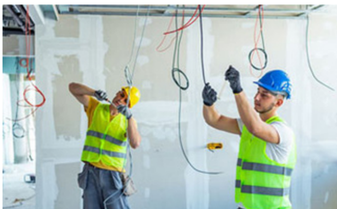
Fig. 1.1.18 Electrician work at site
