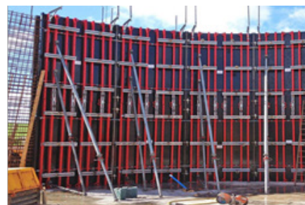
Fig. 1.1.14 System formwork
