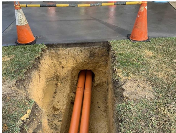
Fig. 3.3.29 Depth of trenches
