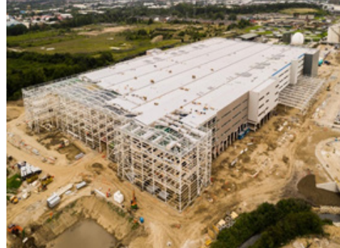
Fig. 1.1.5 Industrial building construction site
