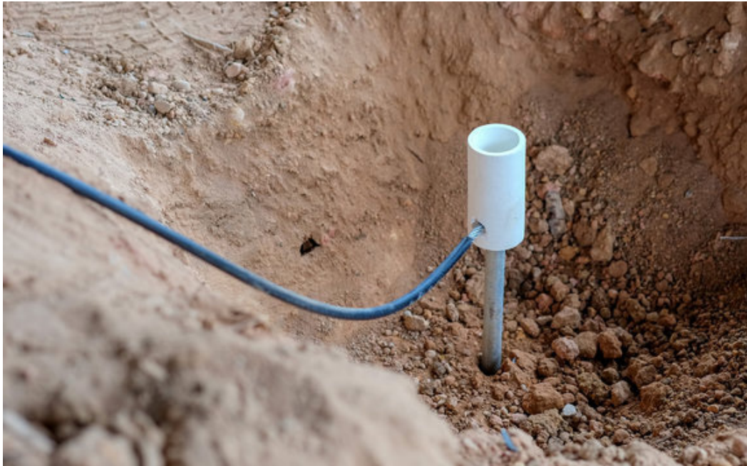
Fig. 3.3.16 Connecting to ground rod
