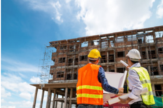
Fig. 1.1.4 Building construction site
