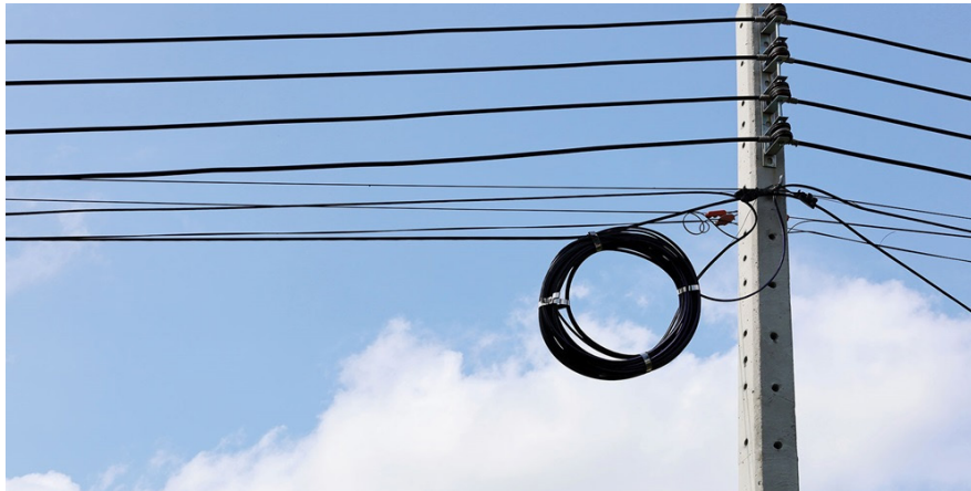
Fig. 3.2.3 Using poles for overhead cable routing
