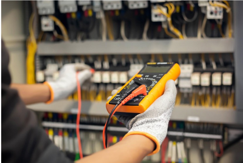
Fig. 3.3.49 Installation and testing of components
