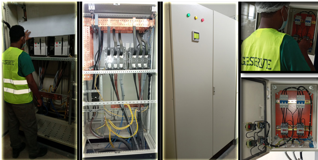
Fig. 5.3.4 Installing distribution boards (DBs)
