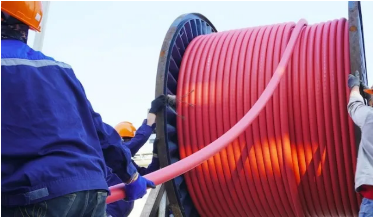
Fig. 3.2.25 Conducting cable laying
