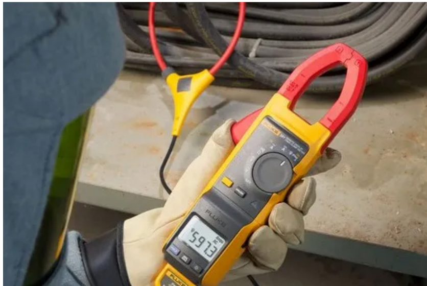
Fig. 3.2.5 Checking the condition of exposed cables
