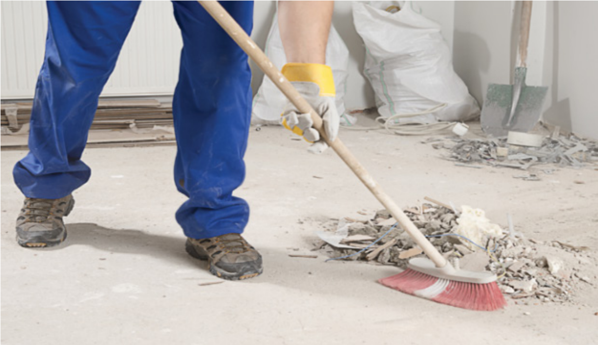
Fig. 8.3.5 Clean-up Debris and Waste
