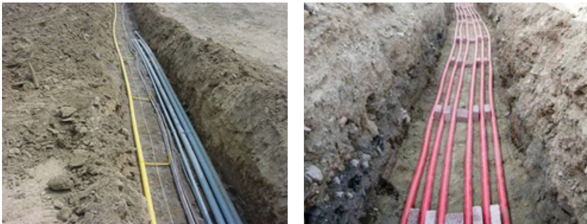
Fig. 3.2.1 Laying cables through trenches
