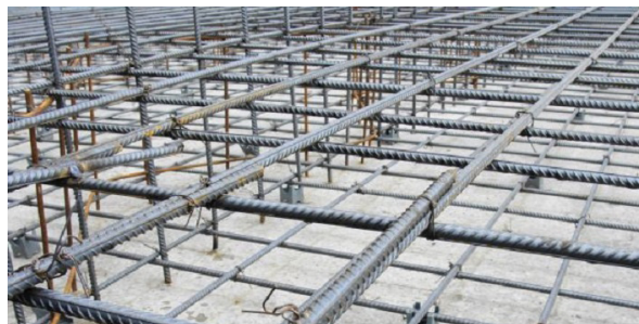
Fig. 1.1.12 Reinforcement bars fixed at site
