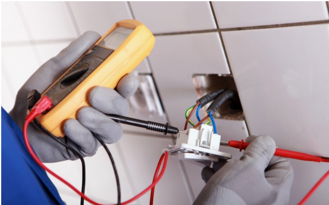
Fig. 5.3.3 Installing electrical fixtures and fittings
