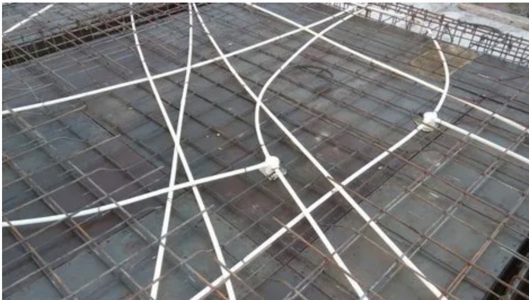
Fig. 5.3.1 Laying flexible conduit pipes through RCC structures
