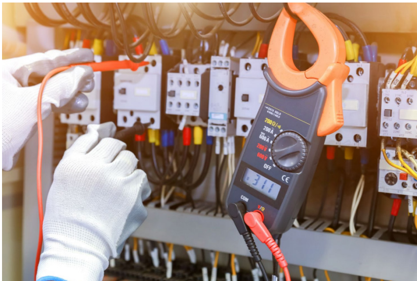
Fig. 5.3.5 Testing connections for continuity and proper wiring
