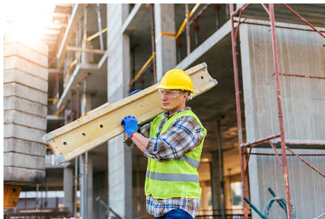
Fig. 8.3.11 Material Handling with Safety
