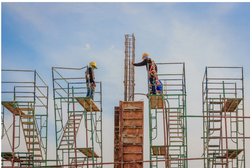
Fig. 6.1.4 Coordination during Construction Work
