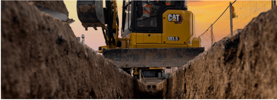
Fig. 3.1.29 Backfilling the trenches with soil
