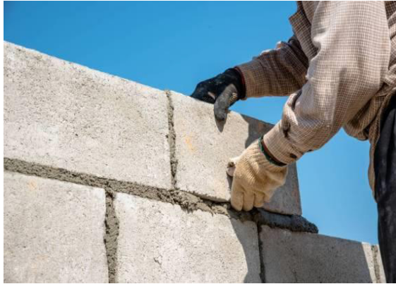
Placing of blocks
