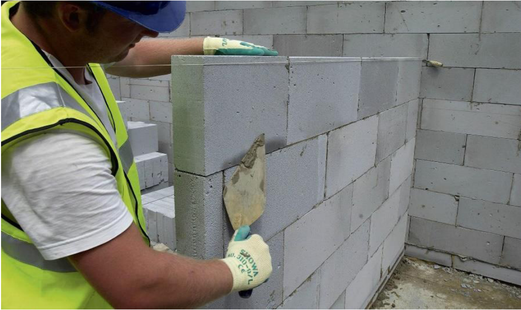
Fig. 4.1.4 Tools used for Block Work
