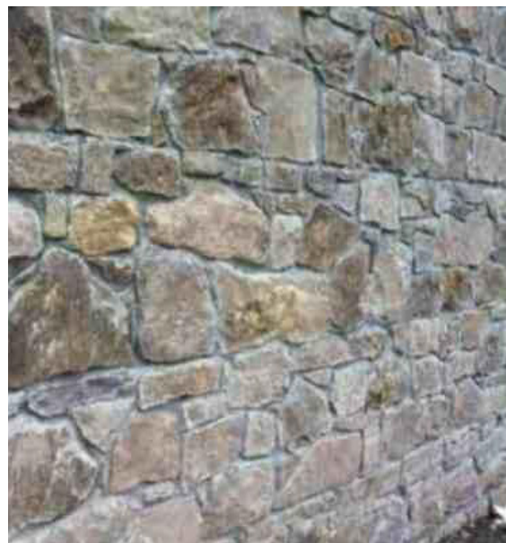
Fig. 12.1.8 Coursed Random Rubble Masonry
