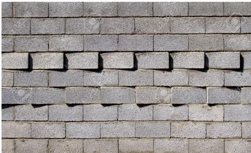
Fig. 4.1.5 Cement Concrete Block Masonry
