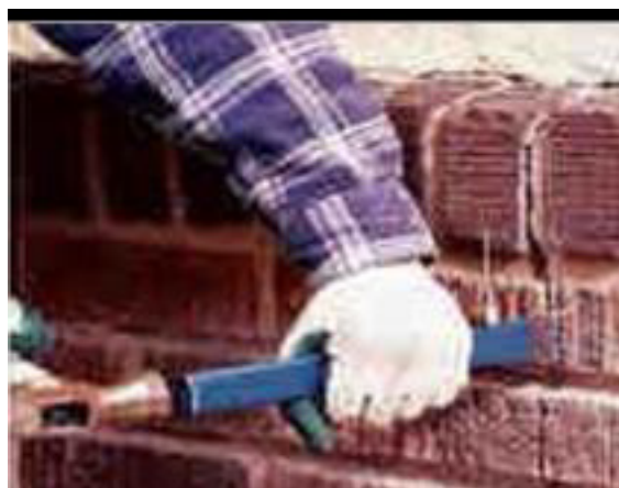
Fig. 3.6.1 Removing of loose mortar
