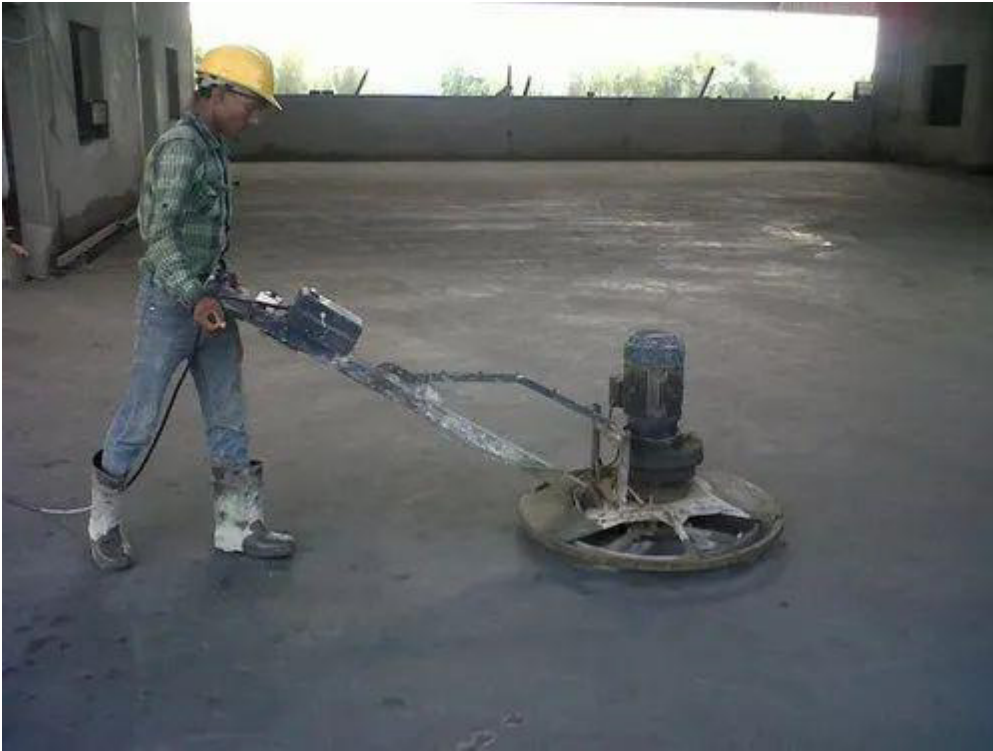
Fig. 11.1.4 Vacuum Dewatering Process
