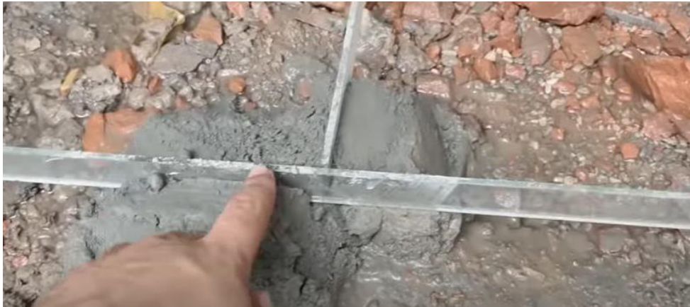
Fig. 9.1.11 Marking dummy dots
