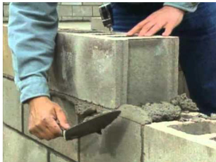
Place the blocks for proper bonding
