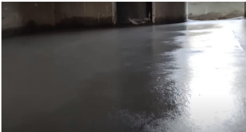
Fig. 9.1.16 Completed IPS Flooring
