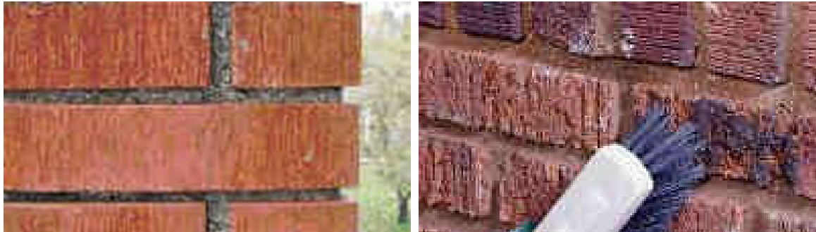
Fig. 3.7.3 Types of pointing
