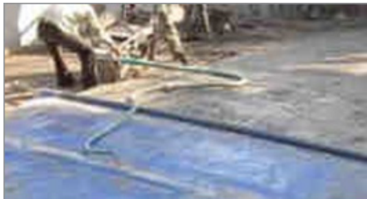
Step 7: Dewatering using the vacuum dewatering system
