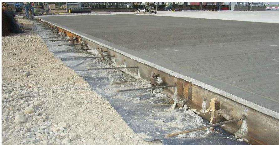
Fig. 11.1.3 Forming of RCC flooring using steel road form
