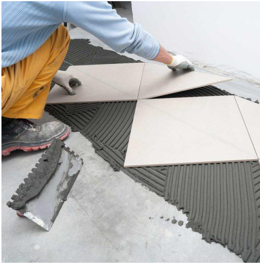
Fig. 6.2.2 Monitoring of Work
