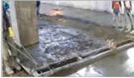
Step 3: Screeding using double beam vibrator
