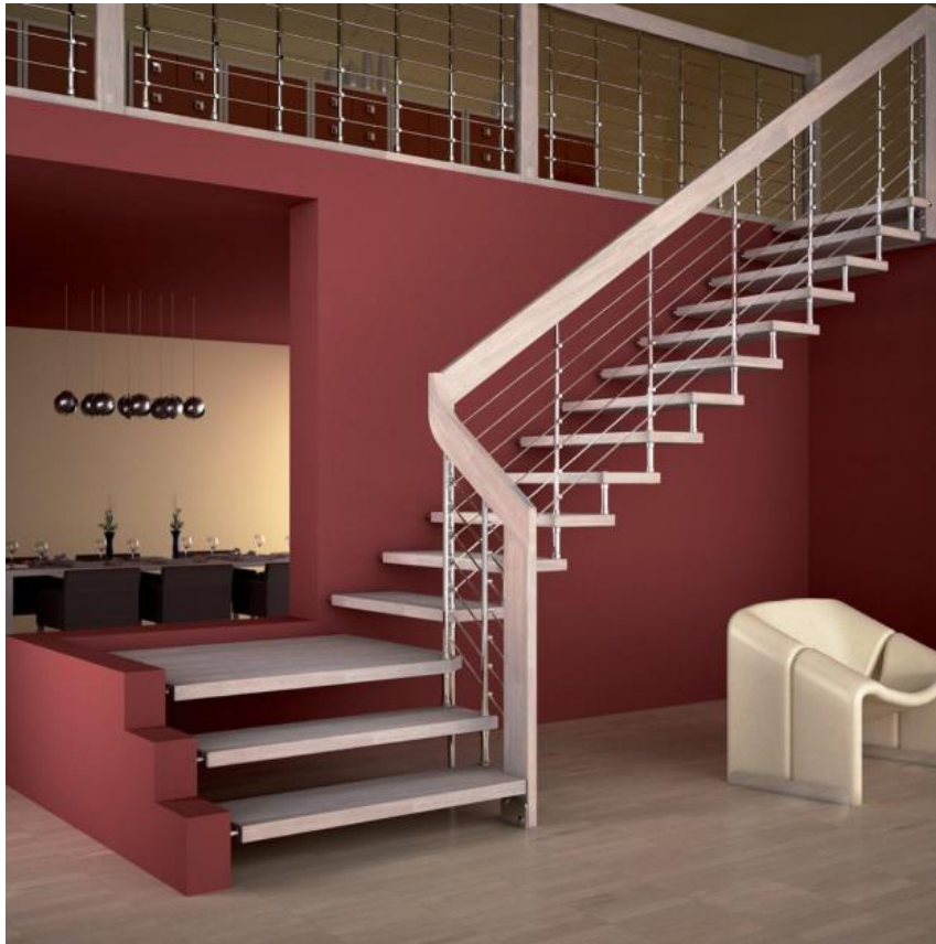
Fig. 3.2.2 Straight run with a single flight and Straight run with a series of flight
