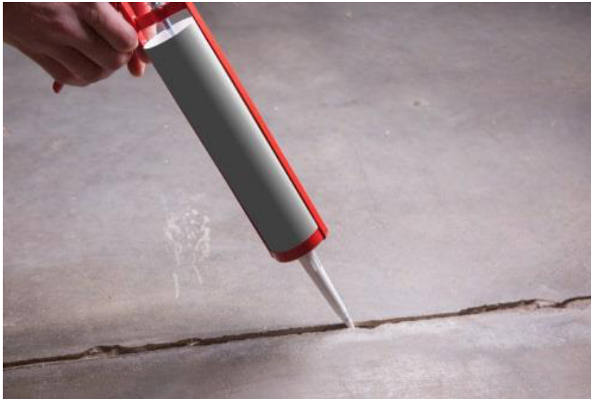
Fig. 11.1.5 Completed IPS Flooring
