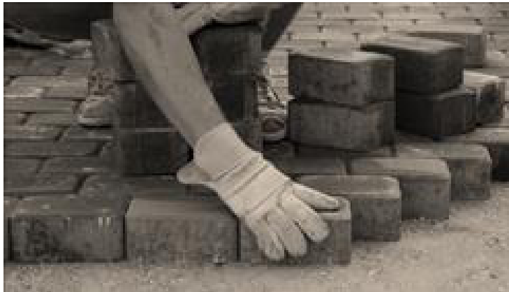
Fig. 3.3.8 Laying pavers blocks
