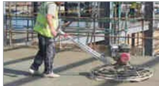
Step 8: Troweling using troweling blades
