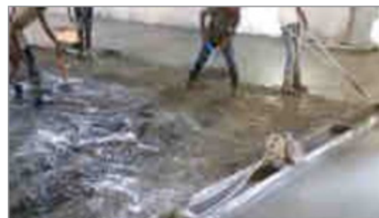
Step 2: Spreading concrete
