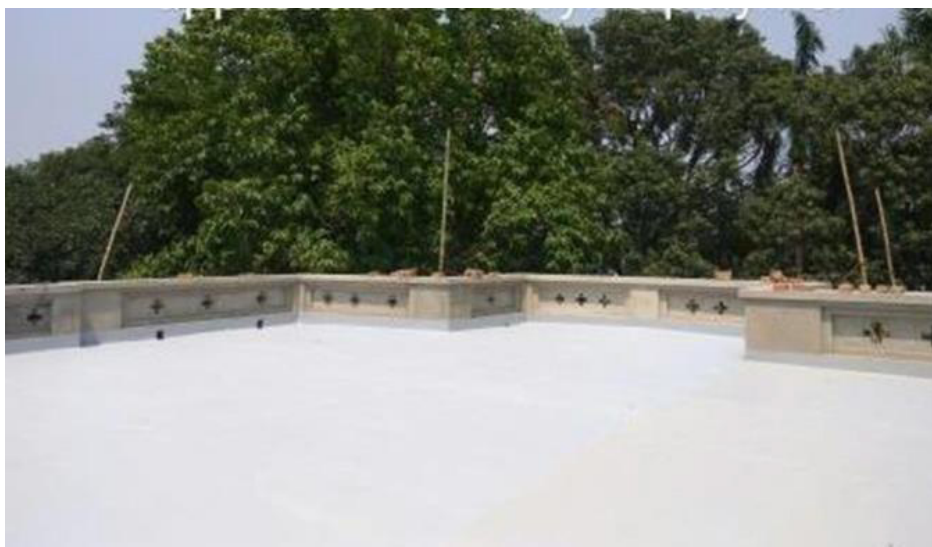
Fig. 8.1.2 Cement / Lime based waterproofing
