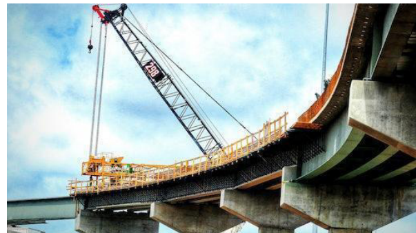
Fig. 1.1.8 Under Construction Bridge
