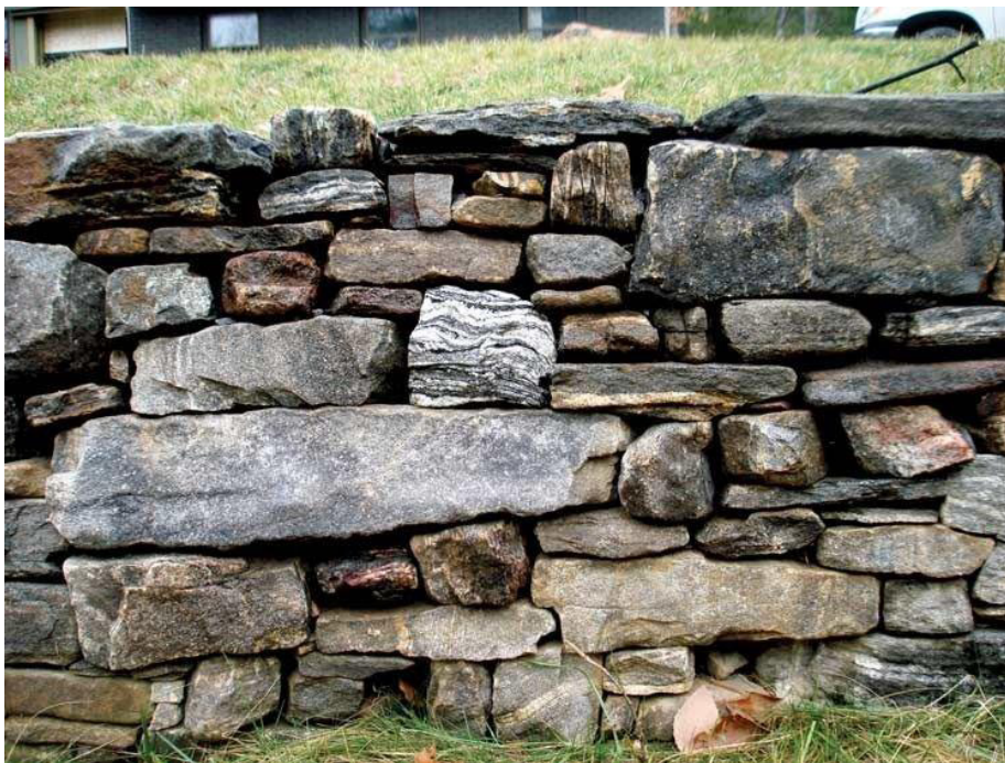
Fig. 12.1.14 Dry Rubble Masonry
