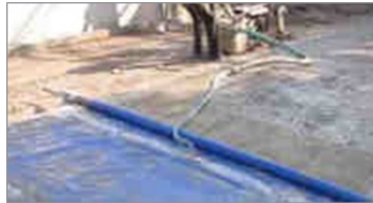
Step 6: Spreading the top cover for dewatering
