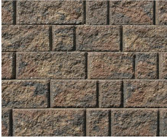
Fig. 12.1.8 Coursed Random Rubble Masonry
