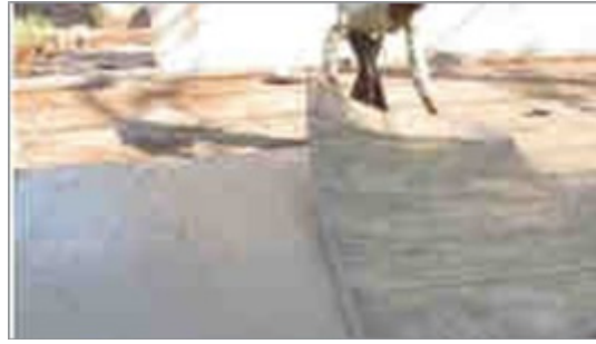
Step 4: Laying the filter pads for dewatering
