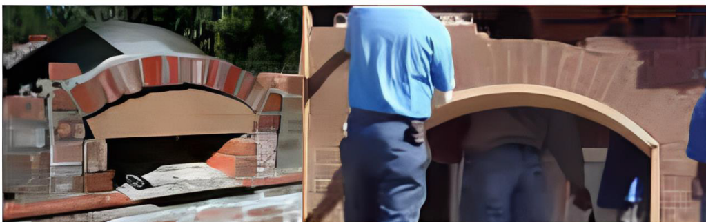
Fig. 3.4.8 Laying Laying of segmented arch
