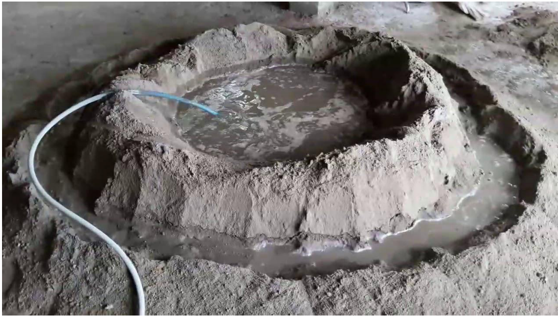
Fig. 8.1.7 Waterproofing Cement Mortar Mixture
