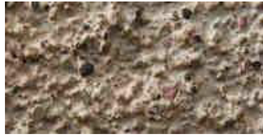
Fig. 10.1.3. Rough Cast Plaster
