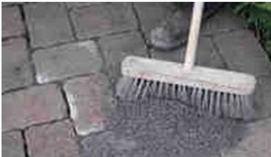
Fig. 3.3.9 Filling joints between pavers blocks
