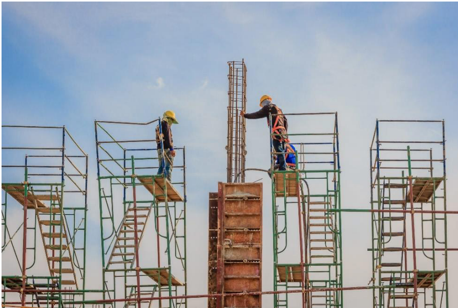
Fig. 7.1.4 Coordination during Construction Work
