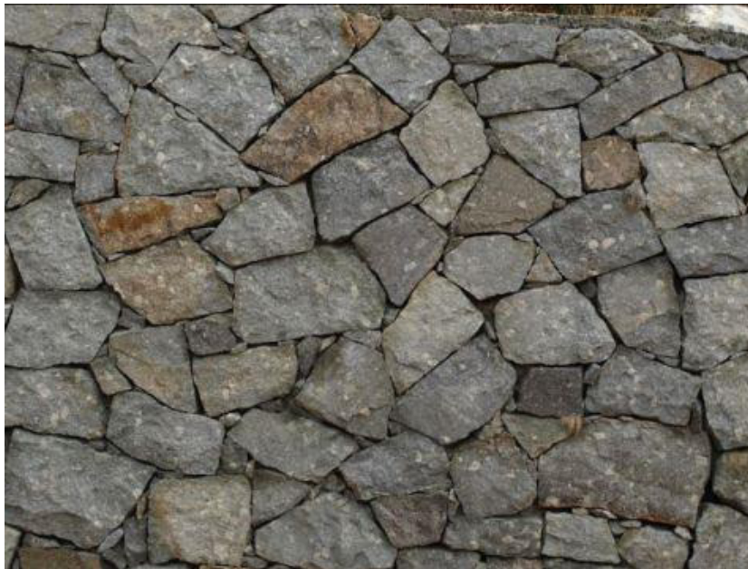
Fig. 12.1.9 Un-coursed Random Rubble Masonry
