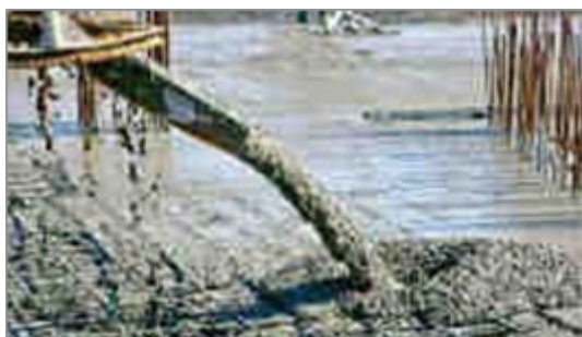
Step 1: Pouring Concrete in the form
