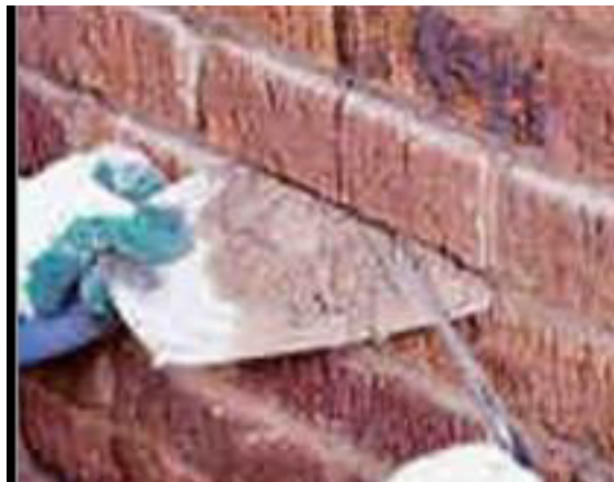
Fig. 3.6.2 Repointing in brick work
