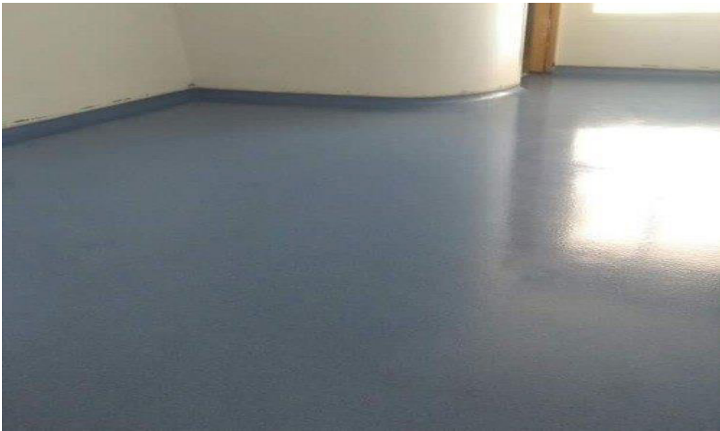
Fig. 8.1.12 Curing the final coat
