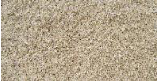
Fig. 10.1.2. Sand faced plaster
