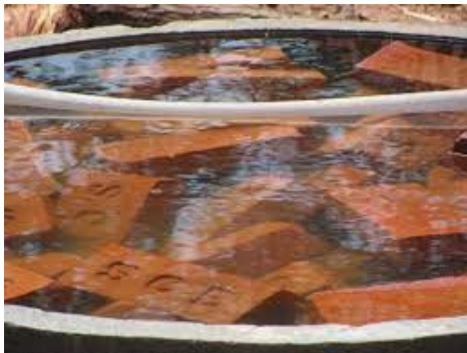
Fig. 8.1.8 Dampening of brick in water
