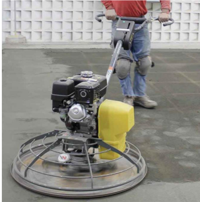
Fig. 11.1.4 Power Trowel Machine
