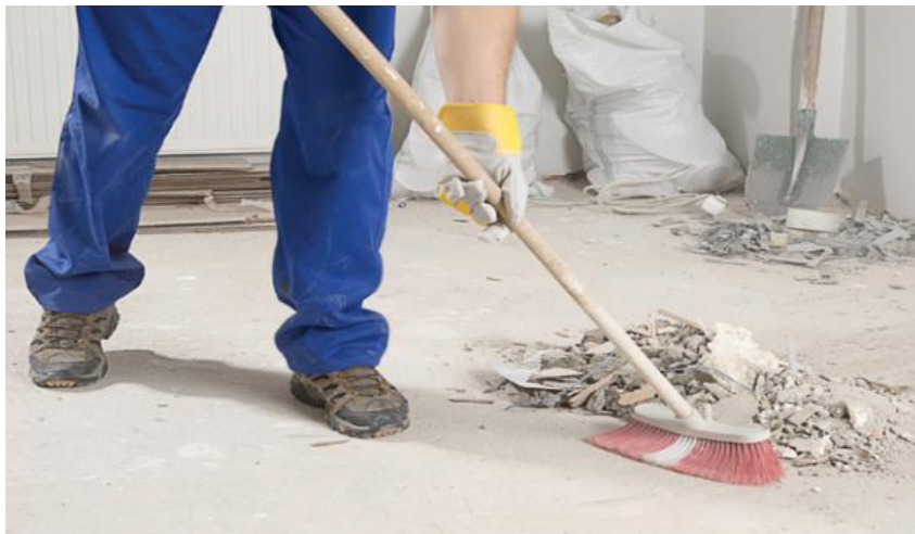
Fig. 5.3.5 Clean-up Debris and Waste
