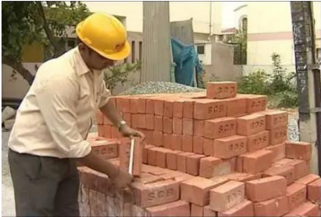
Fig. 3.1.19 Dimension measure of bricks
