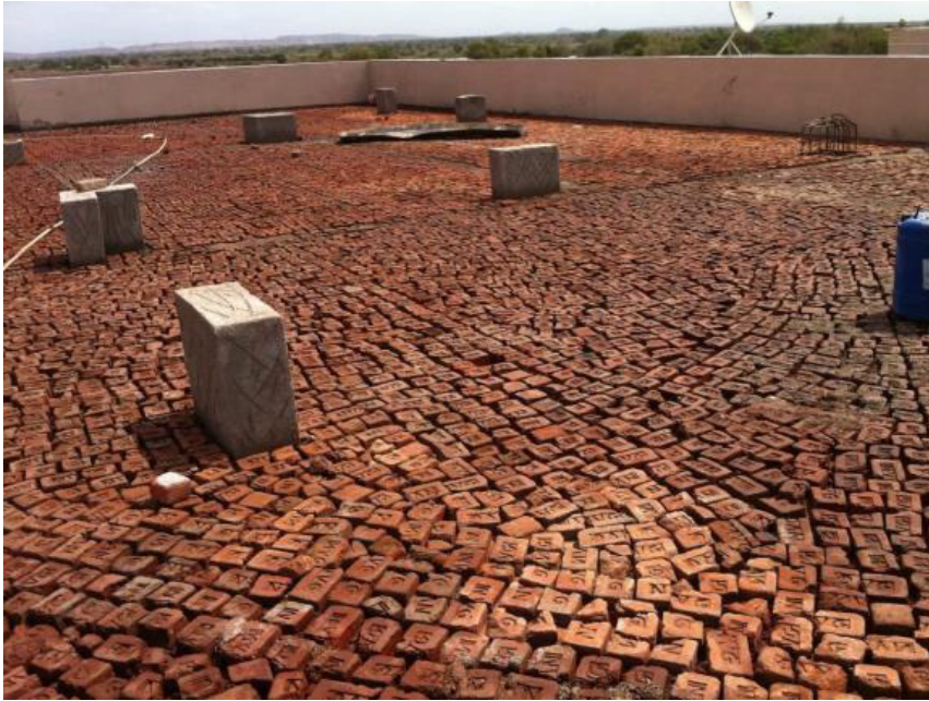
Fig. 8.1.9 Fixing of small pieces
