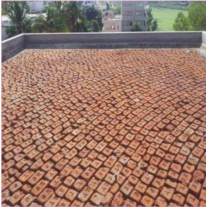
Fig. 8.1.1 Brick Bat Coba Method
