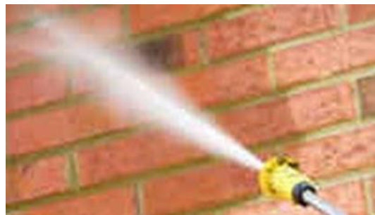
Fig. 3.7.5 Wetting the surface
