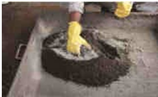
Fig. 12.1.18 Mixing Mortar
