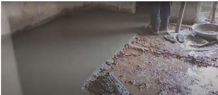
Fig. 9.1.15 Levelling Cement
