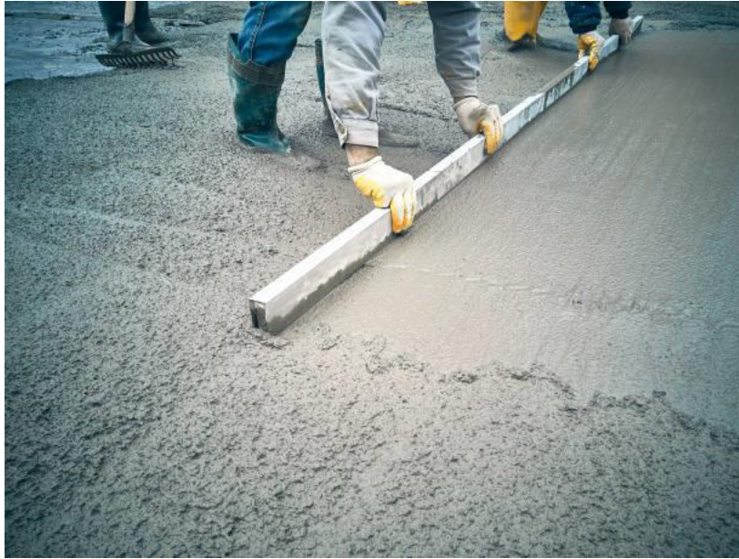
Fig. 8.1.10 Spreading of cement-mortar
