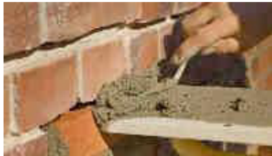
Fig. 3.7.5 Pressing the mortar in the joints
