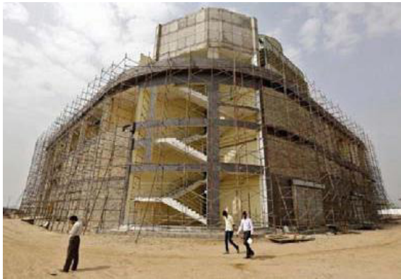
Fig 1.1.3: Building construction site
