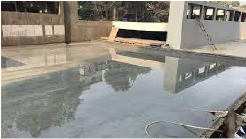
Fig. 8.1.12 Curing the final coat
